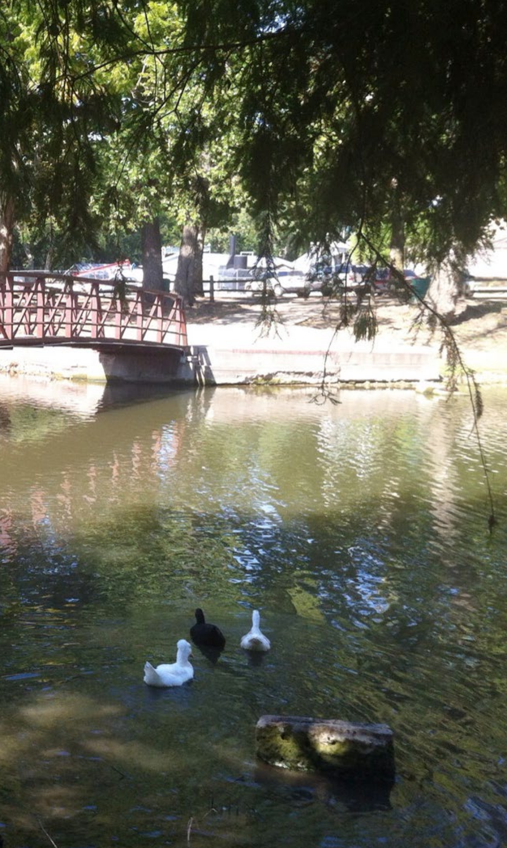
Figure 03: Footbridge in East Park
